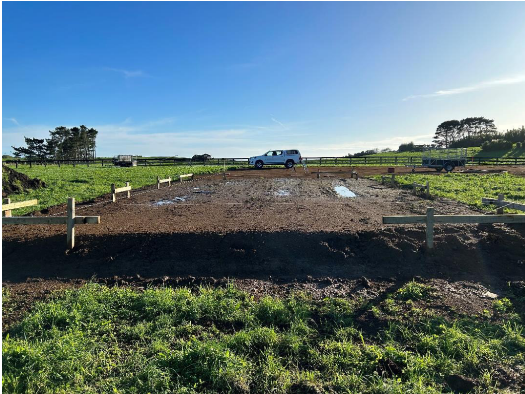
Figure 3.4: Site view facing north, overlooking proposed pole shed platform area. Note that this platform has had earthworks conducted to create a level platform. This is particularly evident at the southern end of the platform, where topography is seen to drop by approximately 0.5 m.
