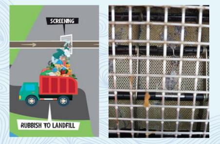
Wastewater first goes through 5mm screens to filter out the large solids in the wastewater, such as wet wipes, rags, food, plastic etc.
