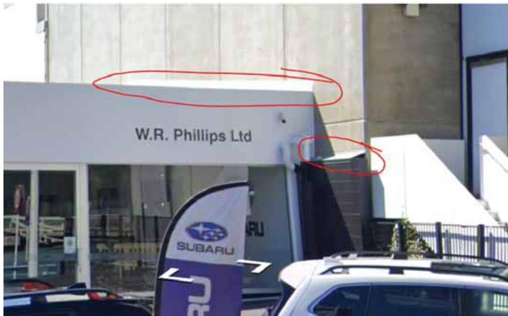
Figure three. The flashings between Len Lye and the showroom
