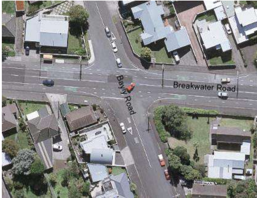
Figure 4-23: Moturoa Suburb Severance
