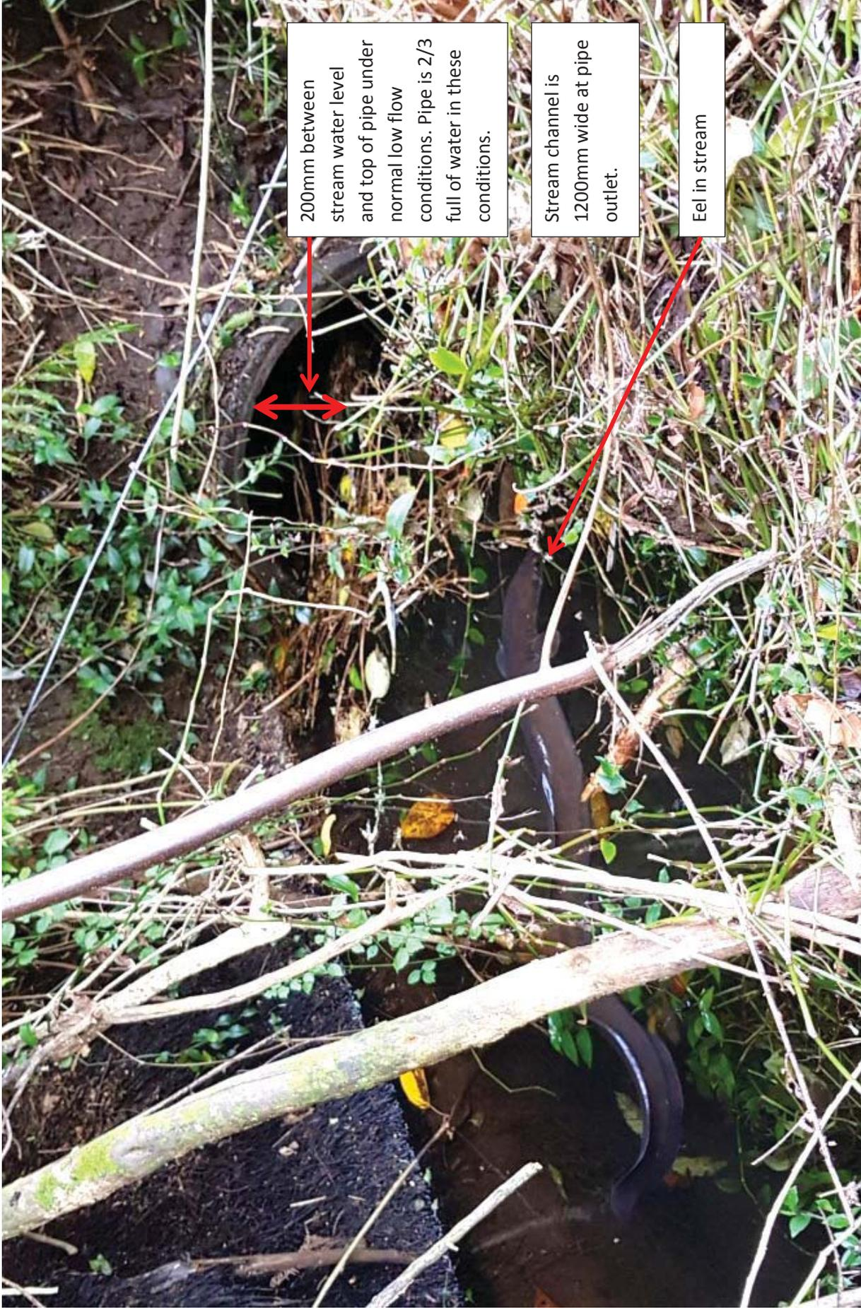
200mm between stream water level and top of pipe under normal low flow conditions. Pipe is 2/3 full of water in these conditions.
