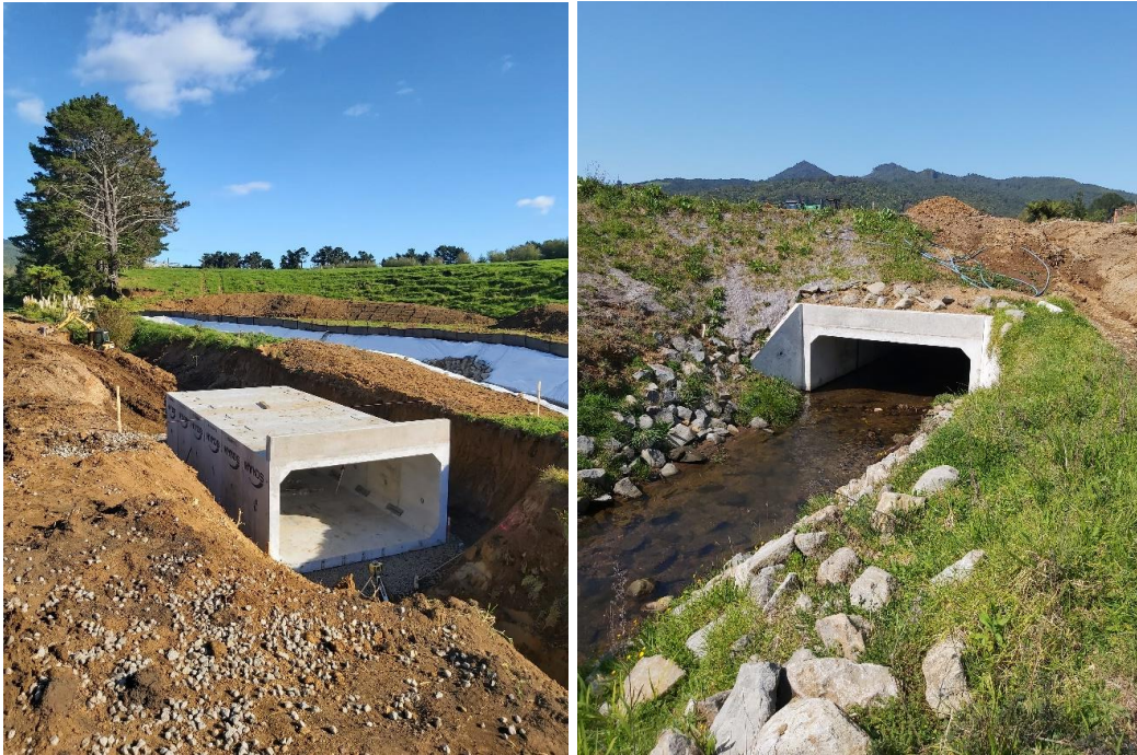
Figure 5: 4m x 2m box culvert
