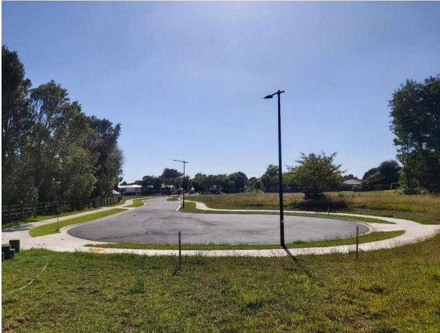
Figure 6: Frankley Road subdivision works progress
