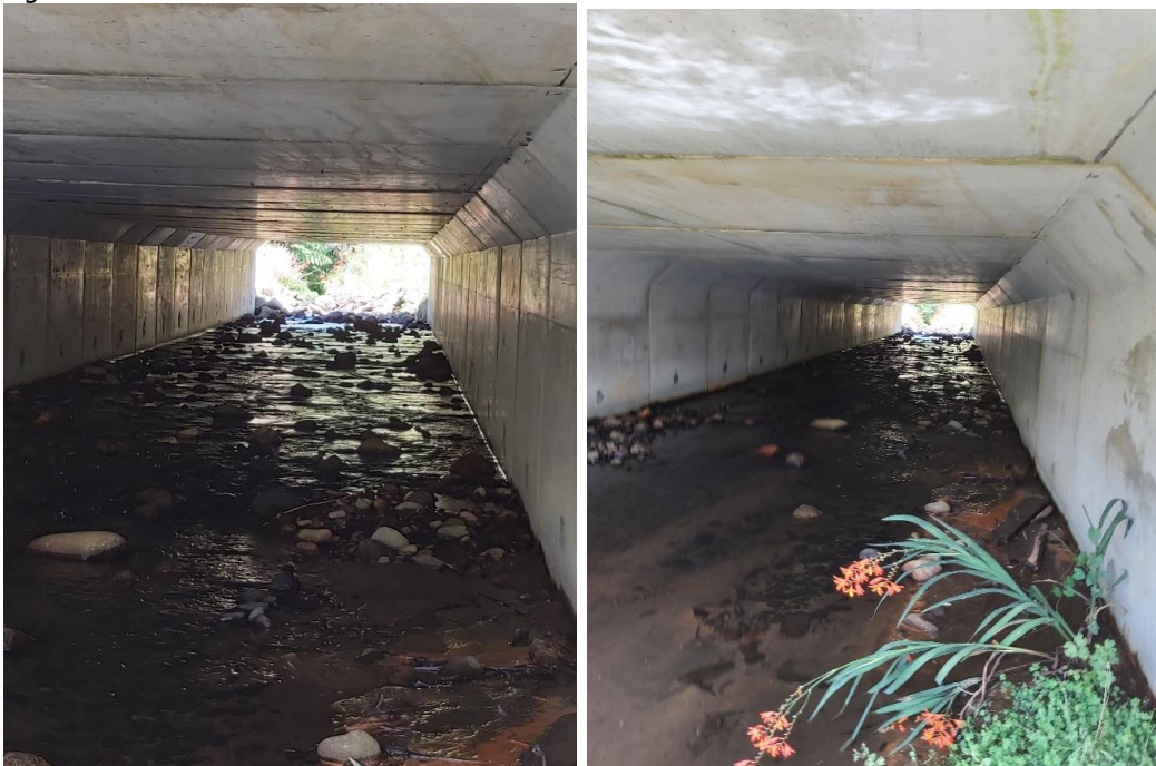
Figure 5: 4m x 2m box culvert
