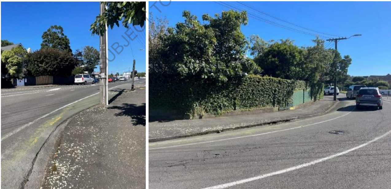
Figure 4-33: Narrow cycleway with fading markings at intersection of Tukapa St and Morley St
