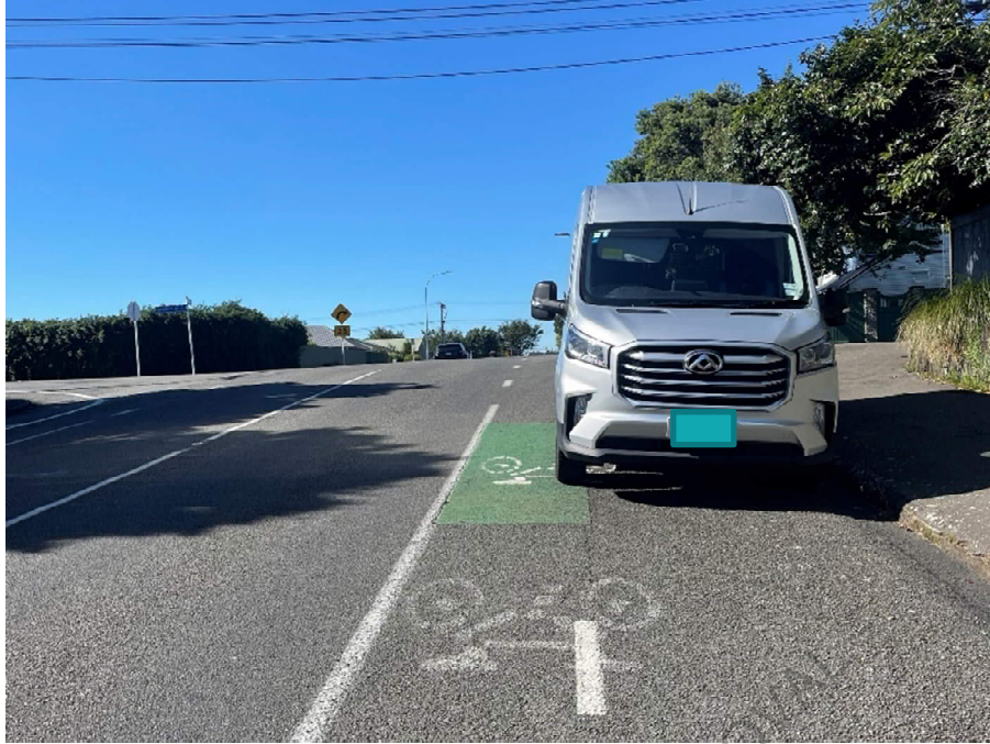
Figure 4-34: Narrow cycle lane at Morley Street
