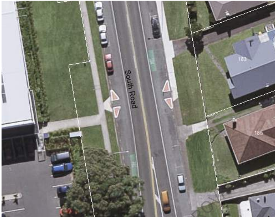
Figure 4-21: Blagdon crossing facilities
