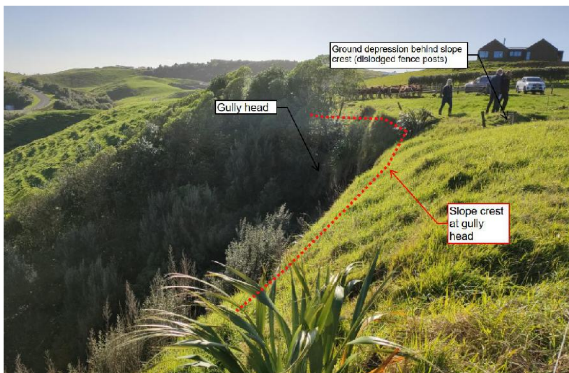
Figure 2.4: View looking north-east at the gully head, slope crest, and ground depression behind slope crest (photo taken during site walkover 4 th August 2021).
