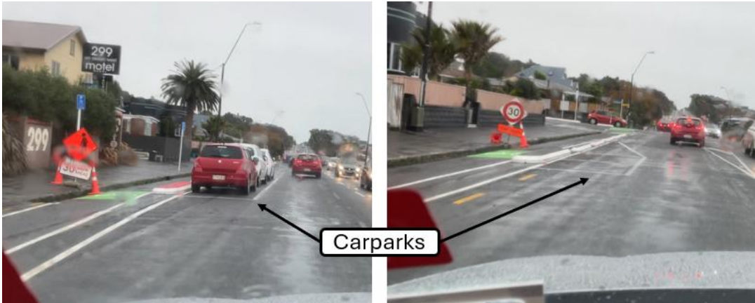
Figure 4-10: Ineffective car park line marking and carparks appearing to protrude into the live traffic lane
