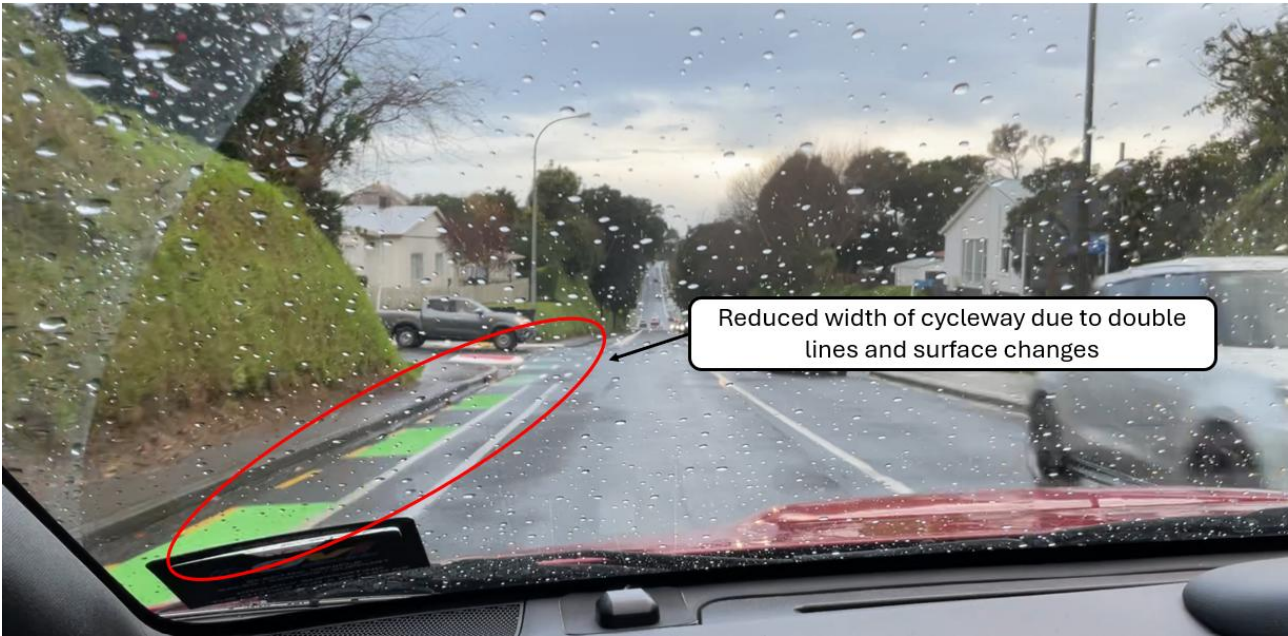
Figure 4-15: Narrow cycleway width caused by line marking, surface changes, and drainage channels
