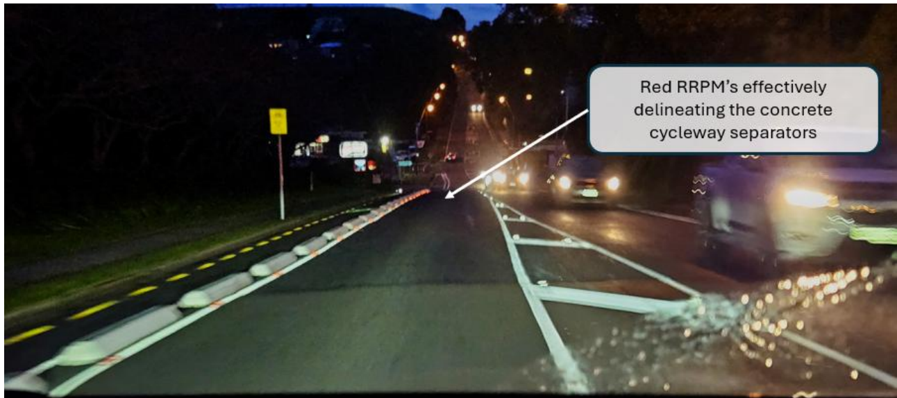
Figure 4-8: Red RRPM's effectively delineating the concrete cycleway separators on SH45 / Devon Street West
