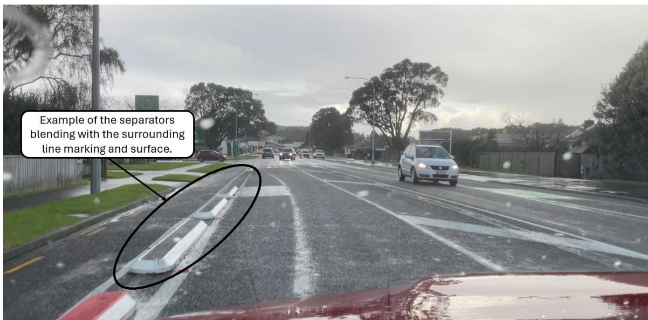
Figure 4-7: Cycleway separators composition matching the surroundings
