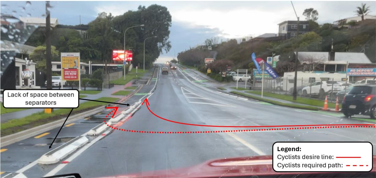
Figure 4-4: Lack of merging space at Seaview Road intersection
