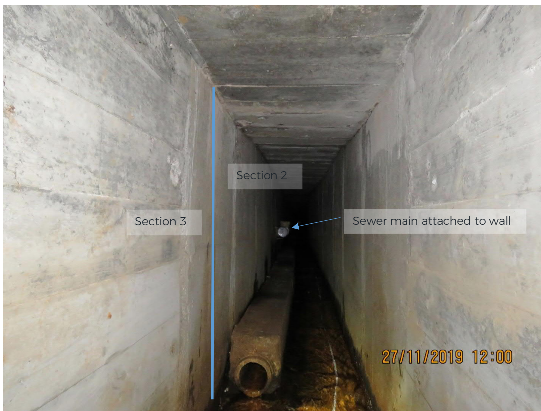
Figure 1-2 : View towards Section 2 looking upstream from Section 3. Note concrete encased stormwater (bottom left) and sewer main attached to true right hand wall.
