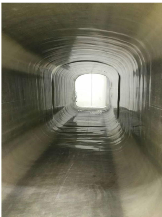
Figure 4-1 : Example cured in place pipe liner
