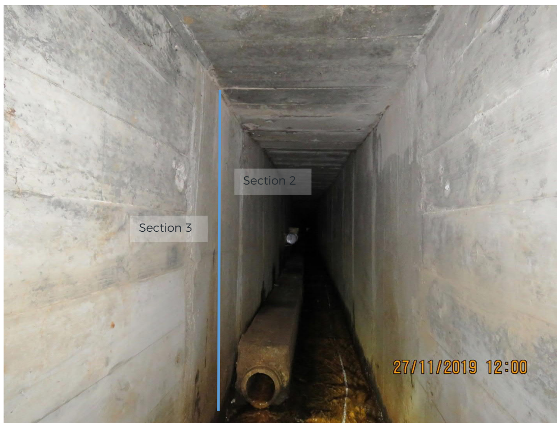
Figure 1-2 : View towards Section 2 looking upstream from Section 3. Note concrete encased stormwater (bottom left) and sewer main attached to right hand wall.
