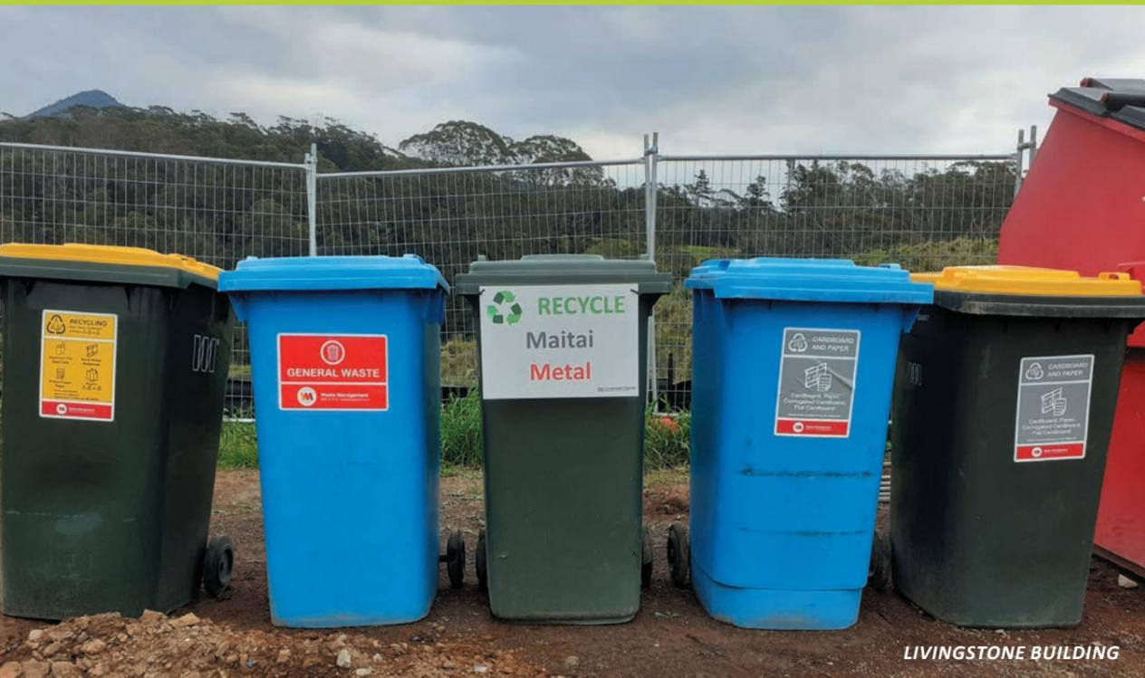
6. Set up separation bins, skips or piles for recycling and reuse, and clear signage for each. A single waste storage area is ideal - many smaller bins over the site encourages people to use the nearest bin to where they're working, and to mix up waste types, leading to contamination and more landfill waste.
