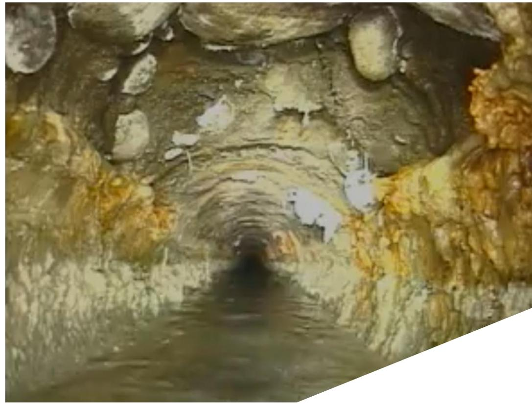
Photo: The soffit of the Connett Road Sewer completely corroded due to H<sub>2</sub>S attack
