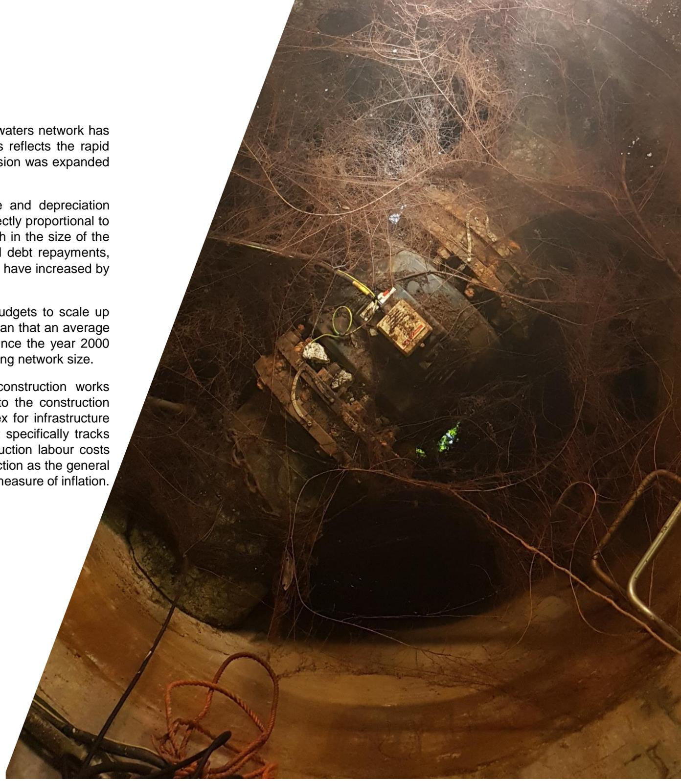
Photo: Tree Root Intrusion in a valve chamber at the Waitara Industrial Water Supply Inlet Works
