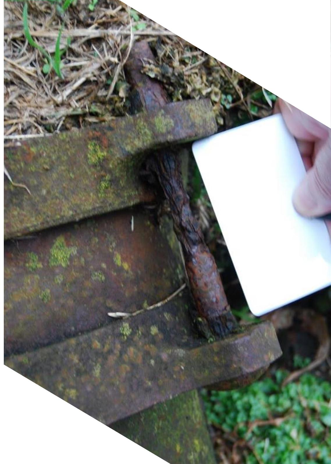
Photo: Corroded pipe joint bolts at the Okato Water Treatment Plant
