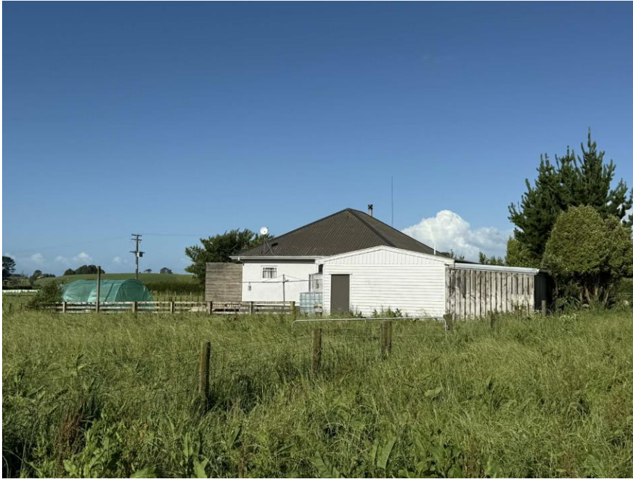
Photo 1: View of the back of the original dwelling, looking from the new dwelling.
