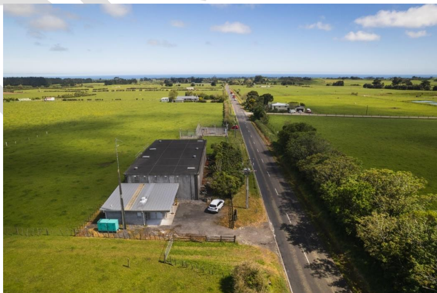
Ōkato Water Treatment Plant
