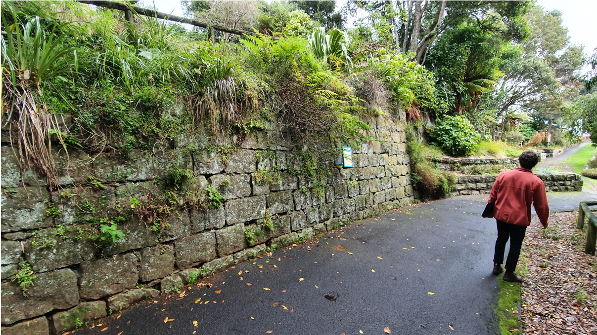
Figure 4: Section of former railway embankment wall, on the opposite side of Powderham Street.
