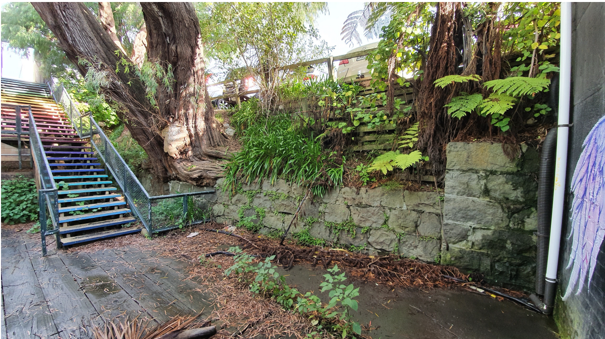
Figure 3: Photograph showing the former railway embankment wall and Agonis Flexuosa .
