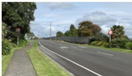
Photo 2 - Close up of 70 km/hr speed limit signs on Veale Road.
