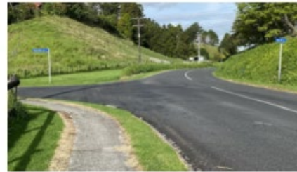
Photo 7 - Close up of Veale Road / Ridgewood Drive intersection. There is a 90 degree left turn into Ridgewood Drive from Veale Road, while Veale Road bends to the right from the intersection.
