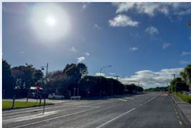
Existing Bell Block Court Road
