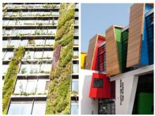
Examples of mitigating building bulk through breaking it up into smaller elements and/or using planting, façade articulation, and/or variation in materials and colour.
