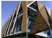
Buildings with good orientation, natural ventilation and shading devices require less energy for heating and cooling while adding to the quality of the building facade.
