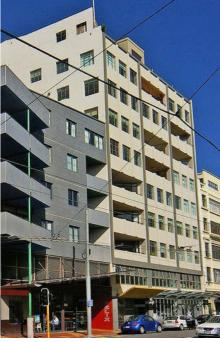
The new building façade to the left is aligned with key façade lines of the adjacent heritage building to the right (e.g. has similar floor to floor height and window size/proportions).
