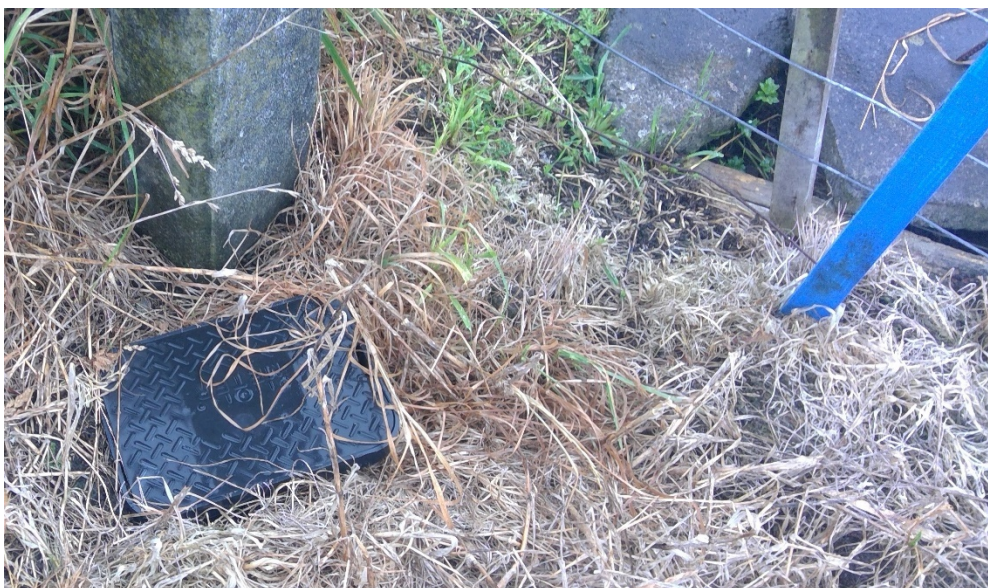
Figure 28: Water connection 24 Te Arei Road West. Image 15 February 2021
