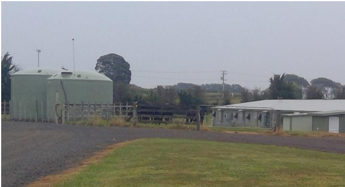
Figure 24: Water tank storage in use Lot 1. Image 15 February 2021
