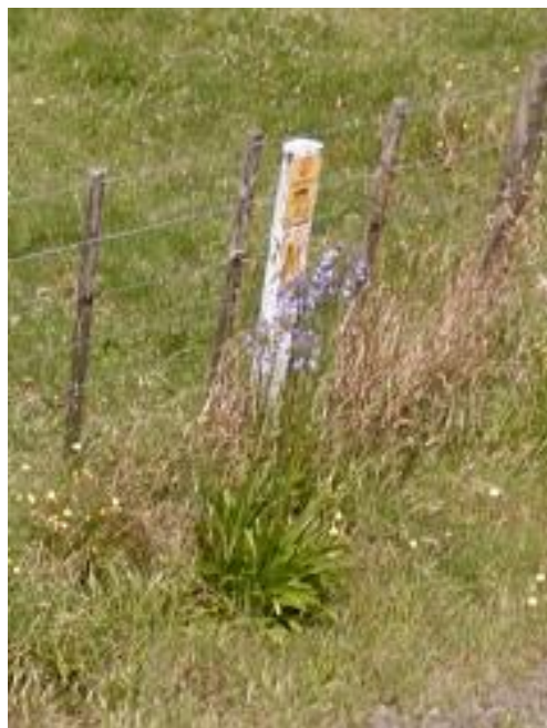
Figure 6: Telco buried sign opposite 24 Te Arei Rd West access point. Image courtesy of Google Maps January 2014.
