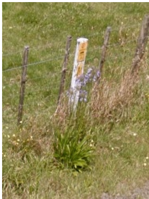
Figure 13: Telco buried sign opposite 24 Te Arei Rd West access point. Image courtesy of Google Maps January 2014.
