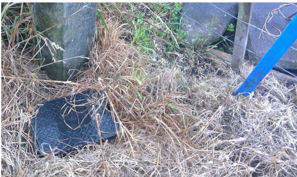
Figure 23: Water connection 24 Te Arei Road West. Image 15 February 2021
