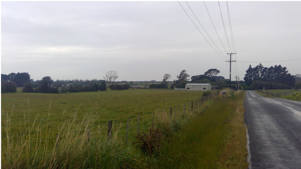
Figure 12: View East from Lot 2. Note: Residential amenity in the form of 11kV Overhead power line, Watermain and Telecommunications embedded in berm. Image 15 February 2021.
