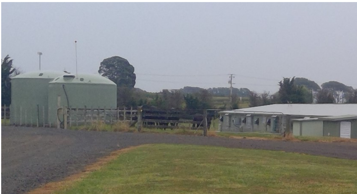
Figure 29: Water tank storage in use Lot 1. Image 15 February 2021
