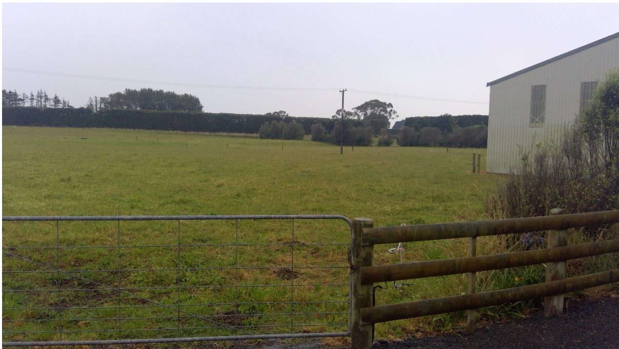
Figure 36: View west over Lots 3 and 4 from ROW entrance. Note tall shelterbelt providing visual mitigation to neighbours to the west. Image 15 February 2021
