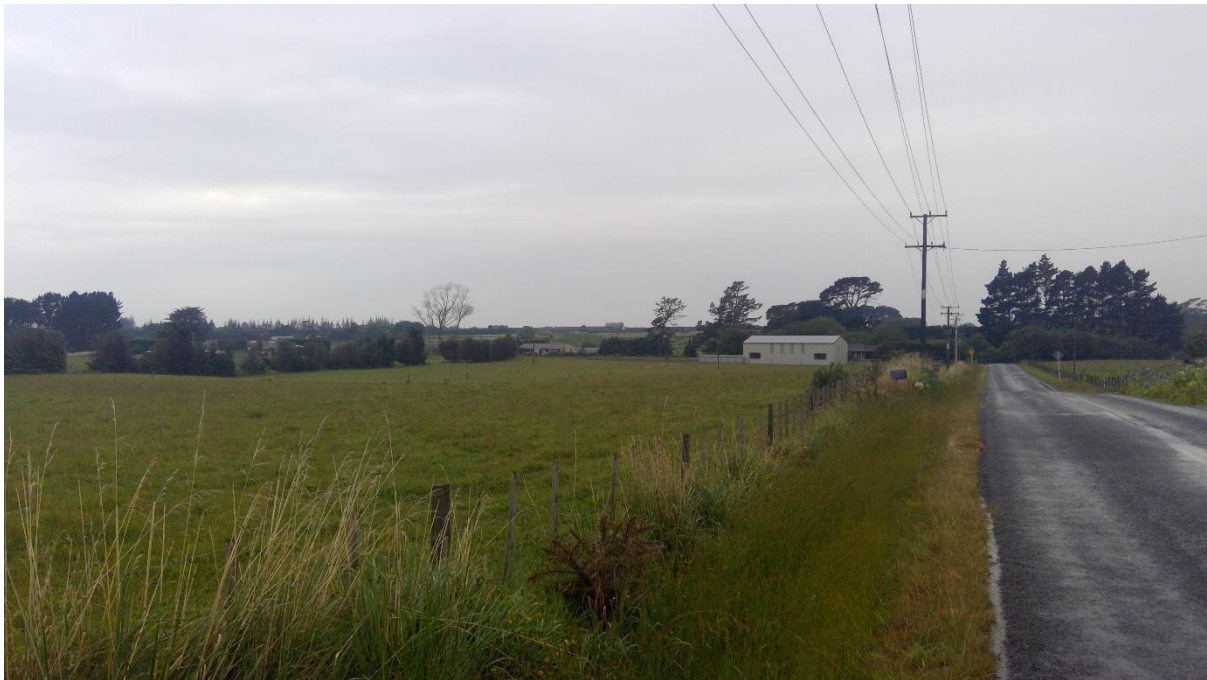
Figure 5: View East from Lot 2. Note 11kV Overhead power line. Watermain runs along berm in left of the road, Telecomm on right. Image 15 February 2021.
